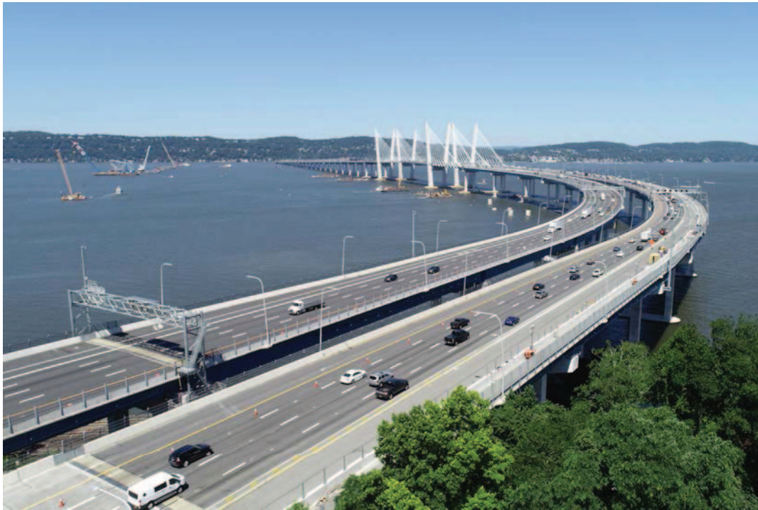
Figure 12: New NY Bridge Project
